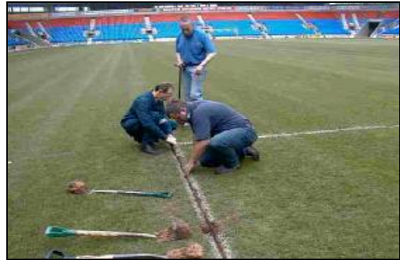
Push sensor to desired depth
